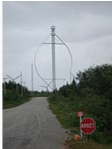
Éole, the largest vertical axis wind turbine , in Cap-Chat, Quebec
